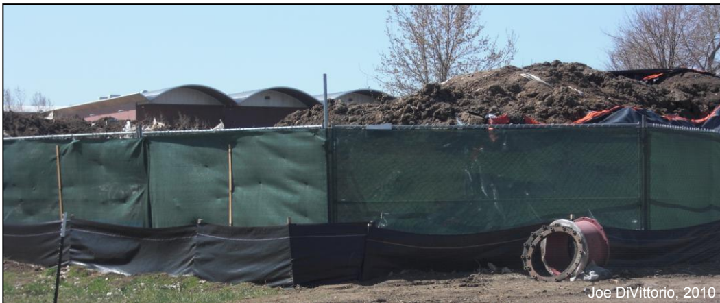
Figure A-4. Stockpiled fill material at a construction site enclosed by silt fencing to help control soil loss and the potential spread of foreign species. Black plastic covering (seen in upper right corner) has been pulled back to allow machine work (photo courtesy of Joe DiVittorio, 2010).
